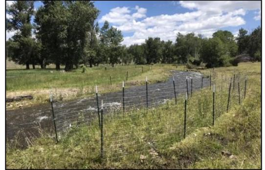
**Miller Creek: Improve the fishery by reducing stream temperatures and sediment delivery.** Partnered with a rancher to install over 3,600 feet of riparian fencing to keep cattle and deer from trampling streambanks and eating new vegetation before it could get established. Planted 400+ native plants and improved natural plant recruitment to help actively revegetate the overly warm, sediment laden stream. *This project reduced sediment delivery to Miller Creek by 19 tons annually.*
