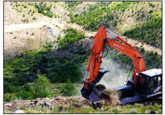
**Rye Creek: Reduce streambank erosion to improve the fishery and reduce excessive sediment delivery to the Bitterroot River.** Enhanced a riparian area using bioengineered bank stabilization, effectively rebuilding streambanks using willows and woody debris, and halting unnatural bank erosion. *Rye Creek is one of the largest sediment contributors to the Bitterroot River; this project prevents excessive sediment from reaching the Bitterroot River.*
